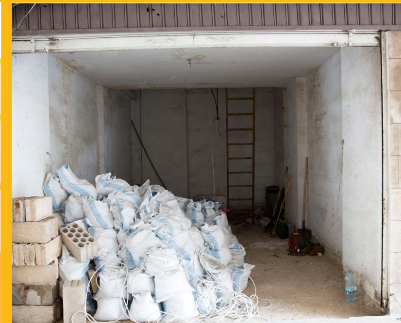
Prayer for All Nations Center - Under Construction
